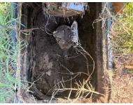
Location of Main Water Supply Valve: Front Side by Meter Static Water Pressure Reading: 47 psi
