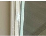
3: Light visible in exterior door weather stripping
