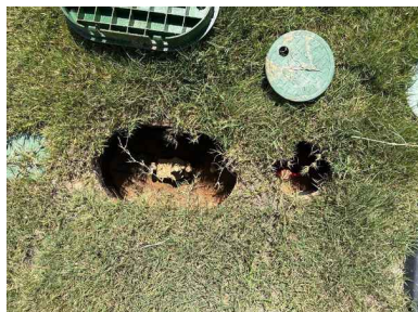
Irrigation backflow and supply valve front, right
