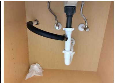
Primary condensate drain upstairs hallway bathroom
