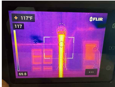
117°F at kitchen sink
