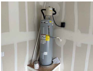
Electric water heater
