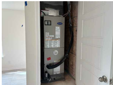
Heat pump, furnace
