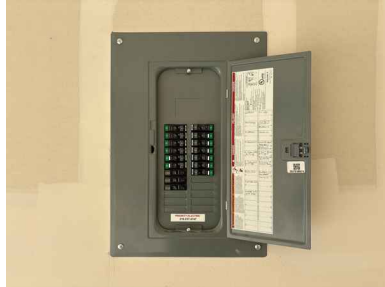
Electrical subpanel
