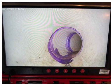
Clean out to rear of home
