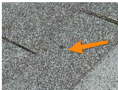
Left side roof face near Ridge
