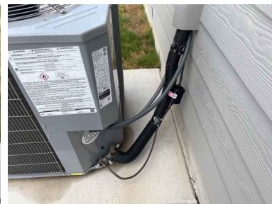
Section line was UV protected and in good condition
